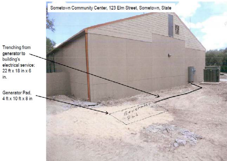
Figure 4. Ground-level photograph showing proposed ground disturbance area.
